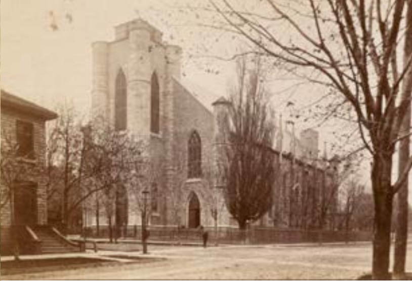
St. Mary's Cathedral Construction of St. Mary's Cathedral began in 1843, but wasn't completed until 1848. Initially the front of the building featured a single belfry, as it did not gain its magnificent tower until the 1890s when Archbishop Cleary undertook an extensive building and decorating program dramatically altering both the interior and the exterior. Queen's University Archives. Henry Henderson Album (F1051-H26)
